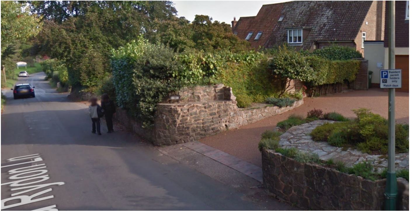
Figure 5: Older existing homes have very poor/zero visibility when exiting driveways onto Old Rydon Lane, having to exit onto the Lane to gain any visibility. This already poses a danger to pedestrians and cyclists when travelling at the edge of the carriageway. Increased traffic along the line will increase this danger by forcing pedestrians and cyclists further to the edge of the carriageway and into the path of cars exiting driveways. The sign in the right of the image also confirms that cars with resident parking permits are legally allowed to park along the Lane, further reducing the already dangerously narrow width.
