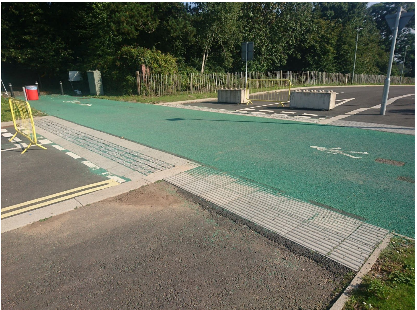
Figure A: Example of pedestrian and cycle priority over vehicles clearly marked where the strategic cycle route on Blackhorse Lane crosses a new access road to the Met Office buildings and car parks at Exeter Science Park.
