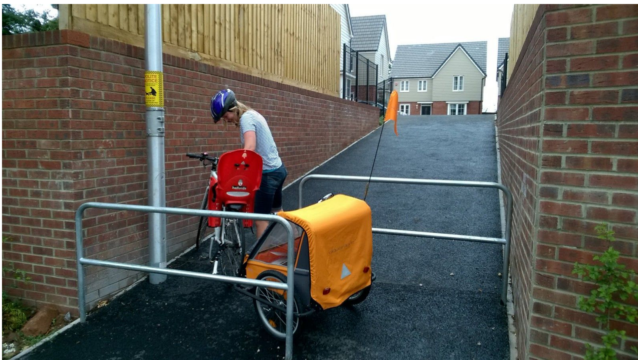
Figure C: Recently installed barriers to cycle path at new development in Newcourt, Exeter. These style barriers are impossible for cargo bikes and adapted cycles to pass through, and difficult for ordinary cycles. They must be avoided.
