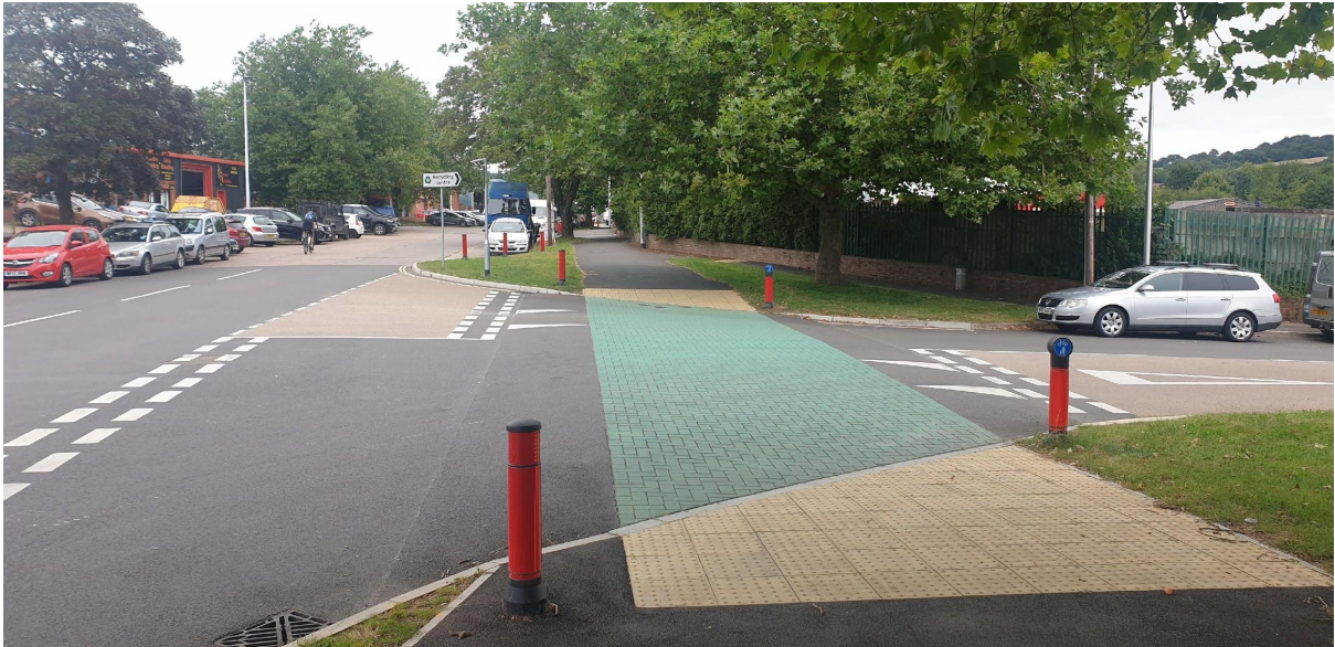
Figure 1 - Pedestrian and Cycle Priority Crossing of side road, junction of Exhibition Way and Pinbrook Road, Exeter.
