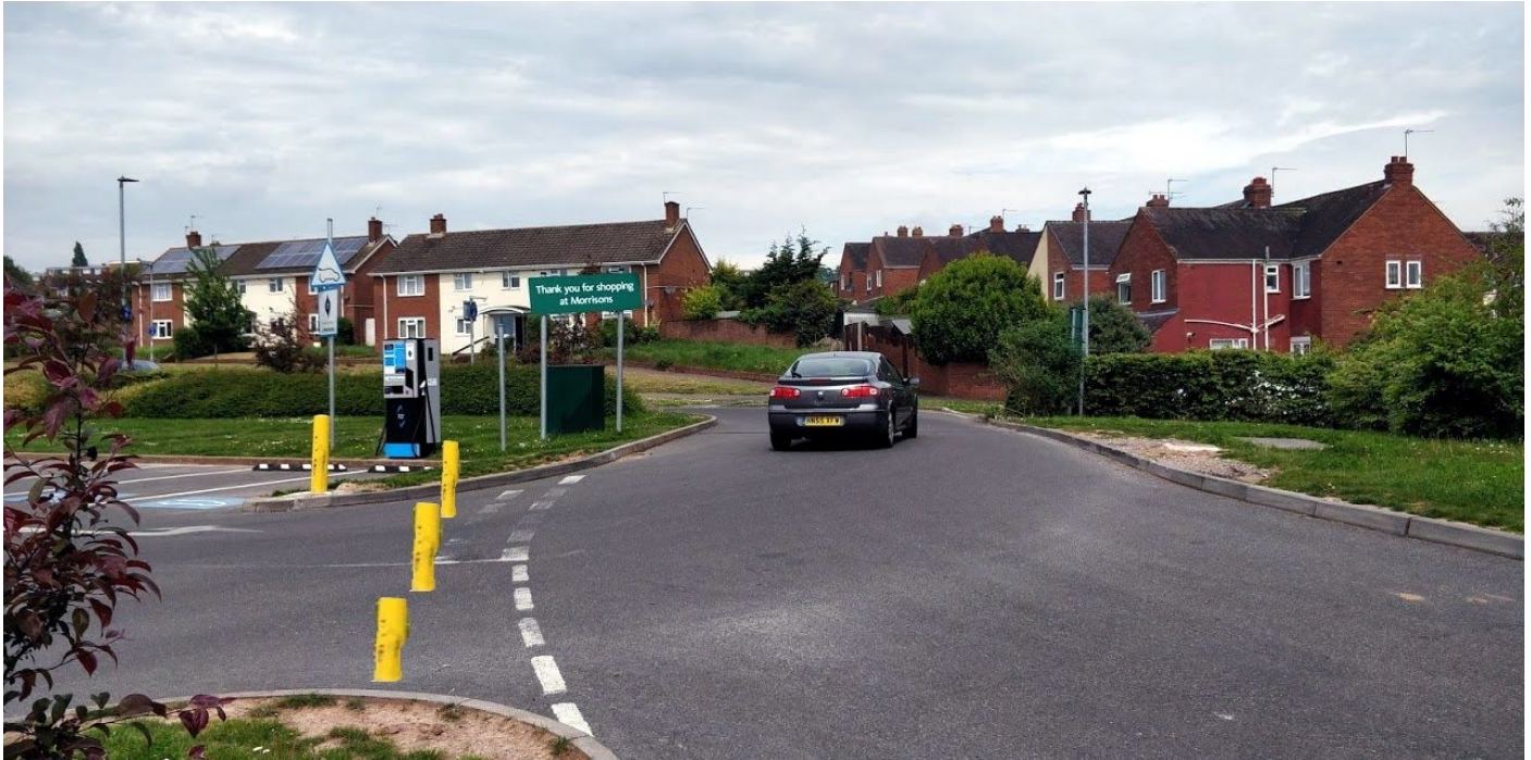
Figure 5 - Bollards. A low cost, practical intervention to improve safety for people walking & cycling
