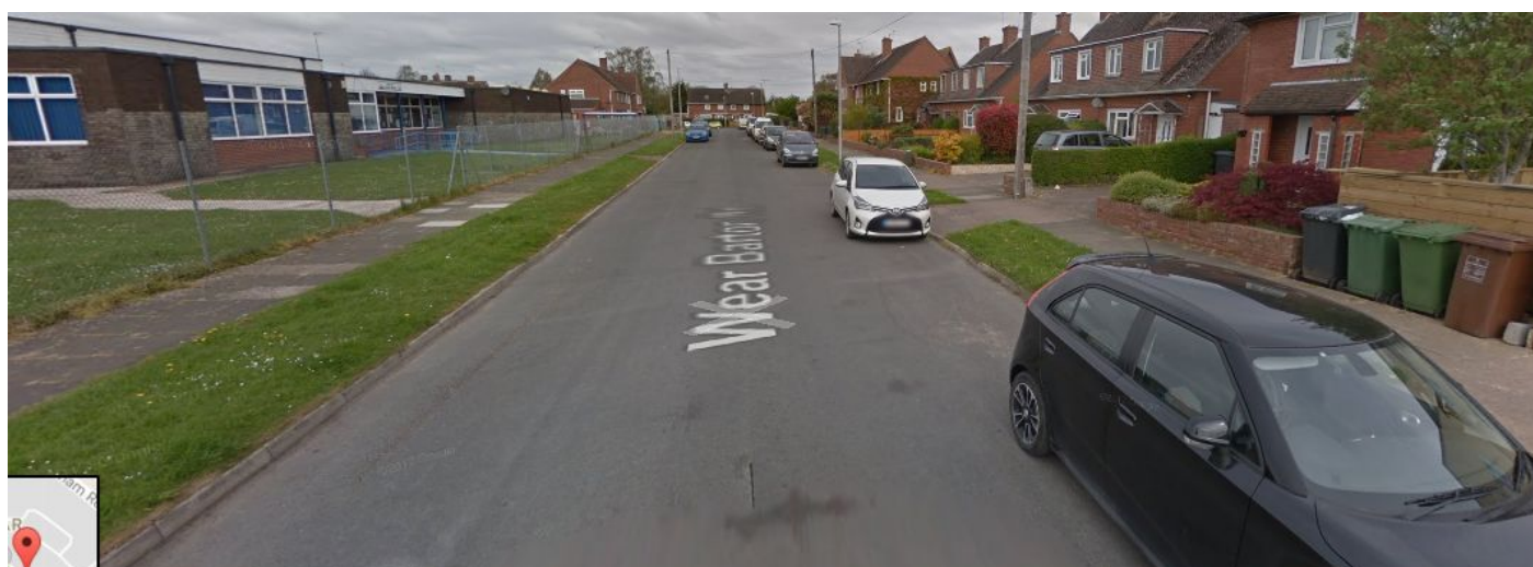
Fig 3. There is space to create separated cycle paths (on the inside of the parked cars) along Wear Barton Lane.
