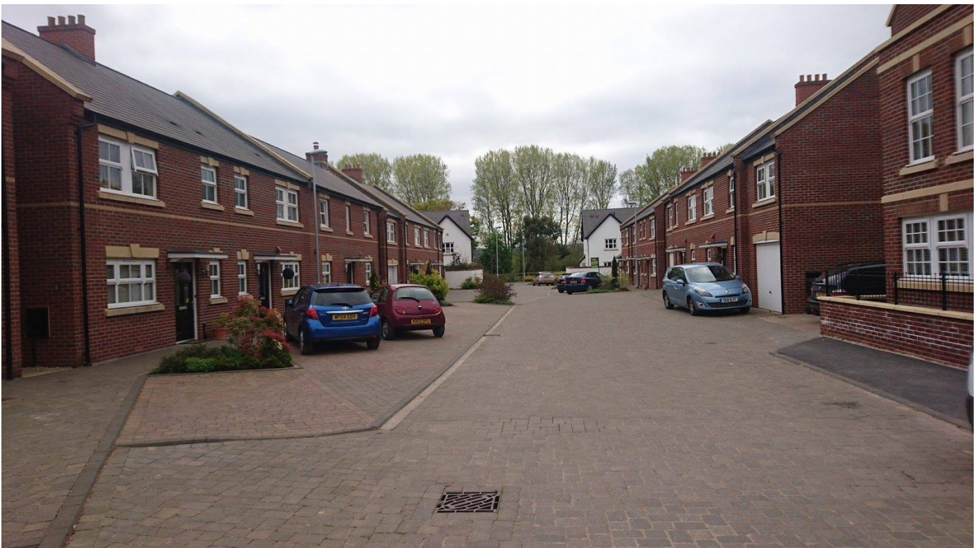
Figure 2b, Millstream, off Topsham Road, Exeter. Pedestrians and cyclists are given equal priority. Vehicle speeds are low due to the lack of defined boundaries. Car parking is perpendicular and delineated through subtle changes in surface colour and through the location of drainage channels and planted areas.
