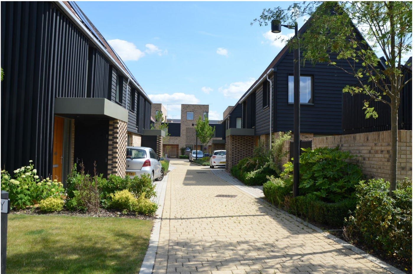
Figure 2a: Abode, Cambridge. Clear priority to pedestrians and cyclists on tertiary streets achieved through narrow carriageway width, use of non-bituminous surfacing and avoidance of kerbs. Car parking is parallel and discrete.
