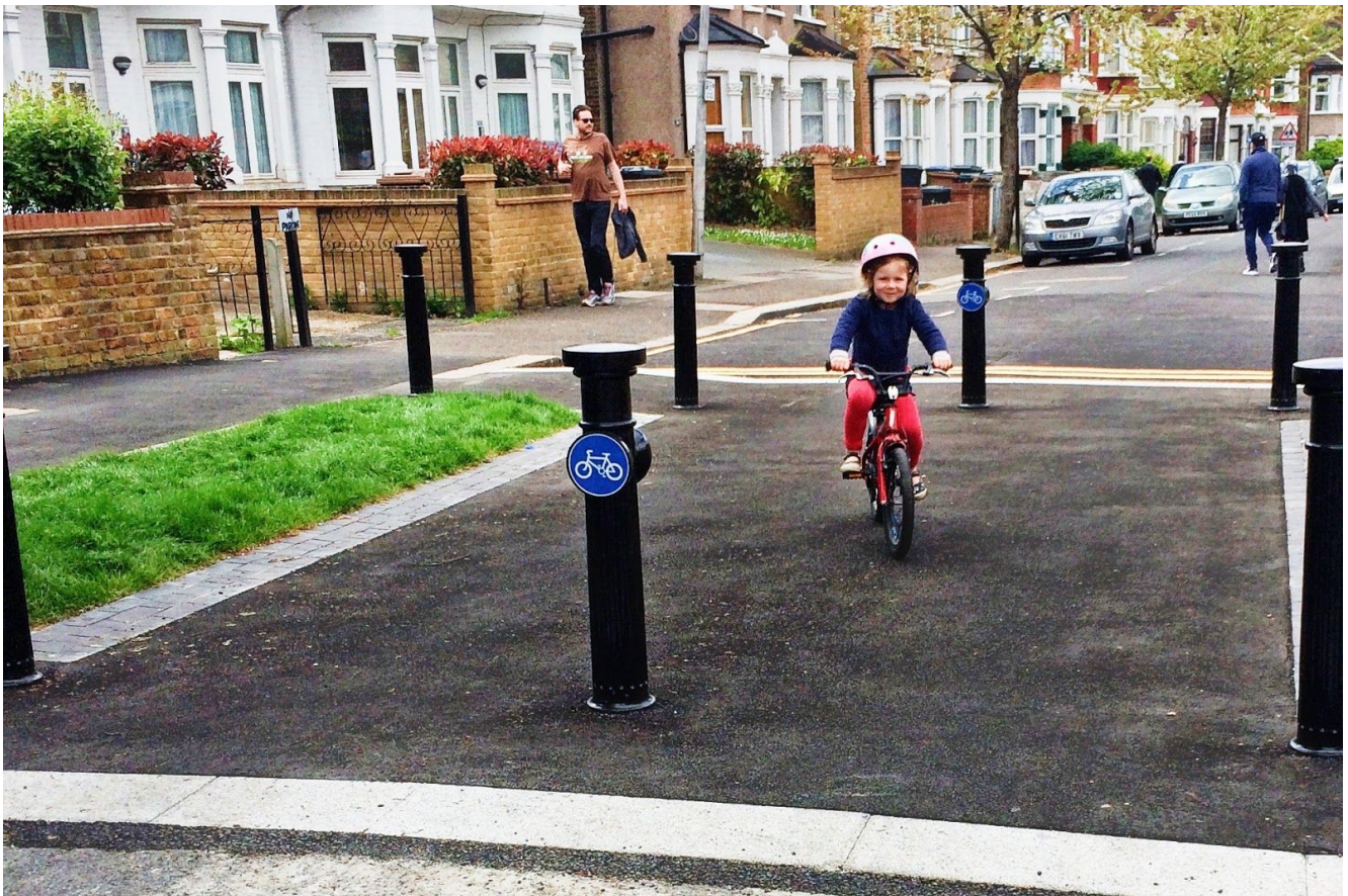
Figure B: Simple bollards with appropriate spacing keep cars out while allowing normal cycles, cargo bikes, tag alongs, adapted cycles and mobility scooters to pass unimpeded. They are also cheap and low maintenance.
