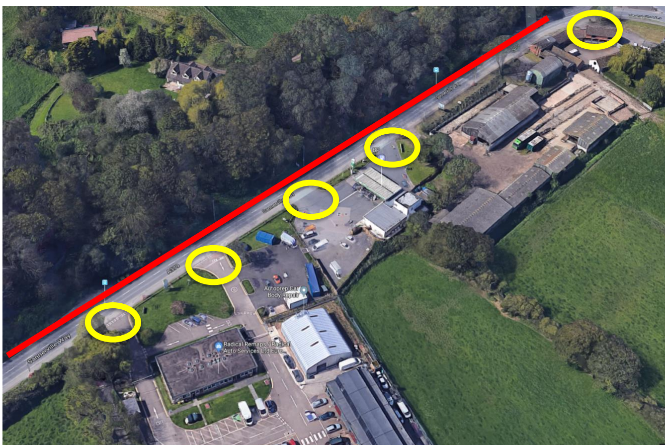
Image 7 – Current shared foot / cycle path along Sannerville Way. Yellow circles indicate the junctions that currently have to be crossed to get between Exminster and the proposed development. The red line shows space on the opposite side of the road where a new cycle path could be installed to provide a direct link to the new development and existing village of Exminster.
