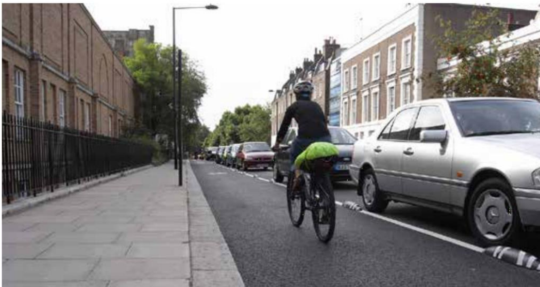
Image 2 – Segregated Cycle Lane, Royal College Street, Camden. Note that lane marking should be on the outside of the raised features. Photo credit to Active Travel (Wales)
